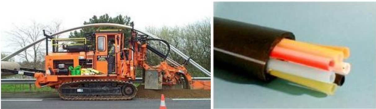
Figure 7: Trenching machine and duct containing multiple subducts
